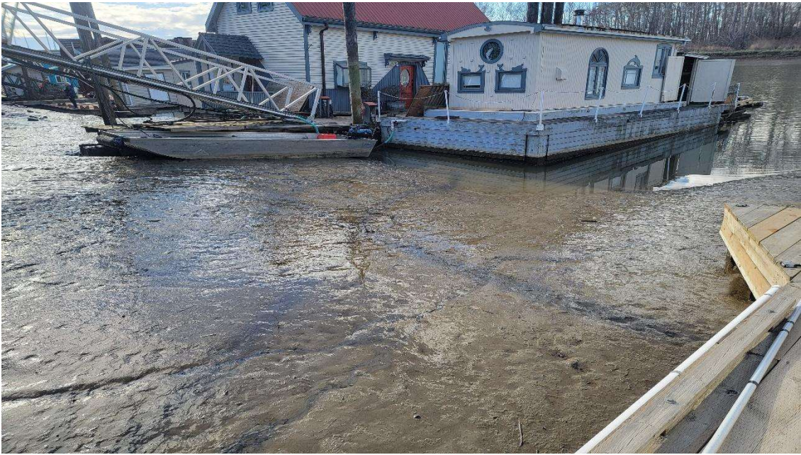
Silt Accumulation within Ladner Harbour
